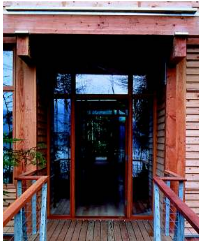
PHOTO 8: Overhangs protect end-grain of beams from moisture.
