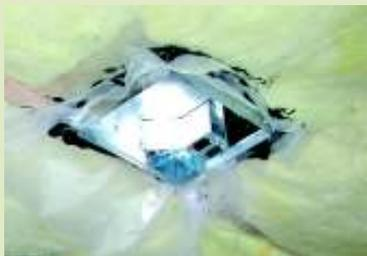
Overlapping of the air barrier, together with caulking around this ceiling air vent, helps to prevent air leakage through the building envelope.
